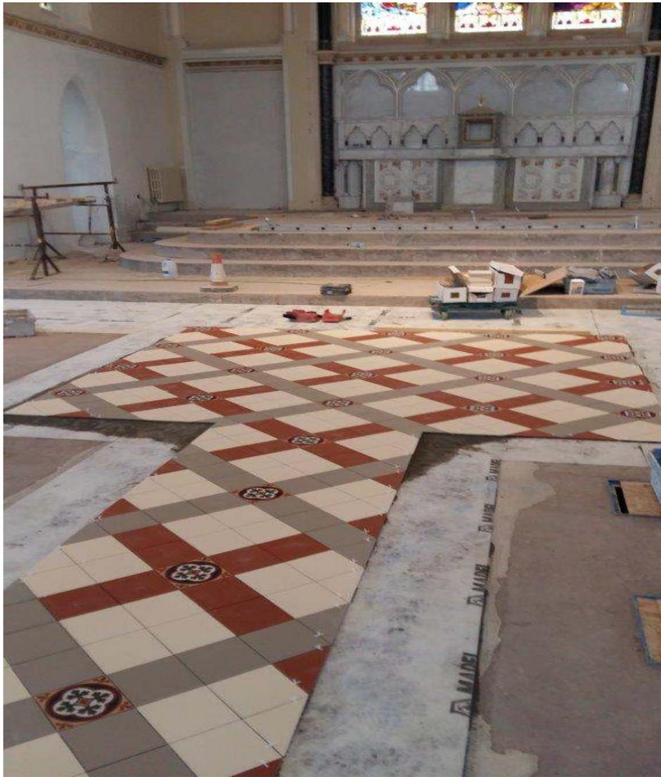
When the old floor coverings were removed damaged floor screeds were exposed. To ensure the long-term structural integrity of the new surfaces Armatile worked in partnership with Mapei to specify products for the contract that would repair the screed and prepare it for the installation of the new tiles. This included installing 225m<sup>2</sup> of Mapei's Mapetex anti-fracture membrane that has been especially developed for problematic substrates.
