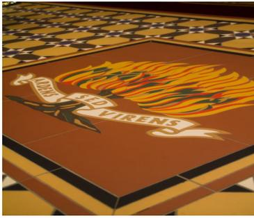
The client wanted a special crest, The Burning Bush, made and installed. Using a photograph of the Burning Bush on the Pulpit Fall, Armatile designed, programmed and manufactured a one off panel for this project.
